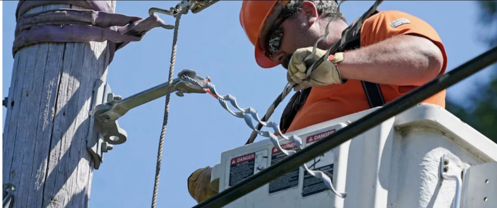
Travis Sheetz, a worker with the Mason County Public Utility District in Washington, installs fiber optic cable on a utility pole while working with a team to bring broadband Internet service to homes in a rural area. (Ted S. Warren/AP)
